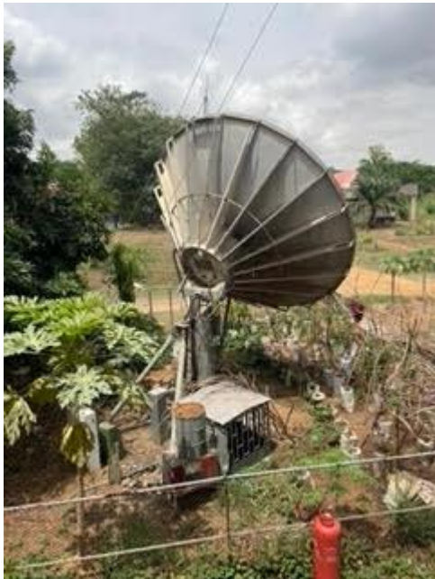
Here is a satellite dish outside a prestigious office block. (Notice the tree nursery to the right and the pawpaw tree to the left.) Wifi and the power supply are constantly switching off, so generators are to be seen and heard everywhere.
